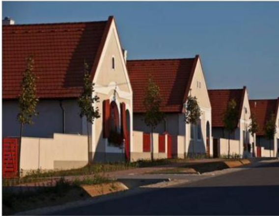
Fig. 13 New houses in the most affected village, Kolontár [26]
