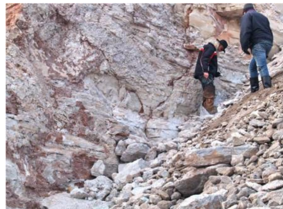
Fig. 6 Western wall having removed the fresh surface of the break. Open fissures with dislocations of a size of dm [10]
