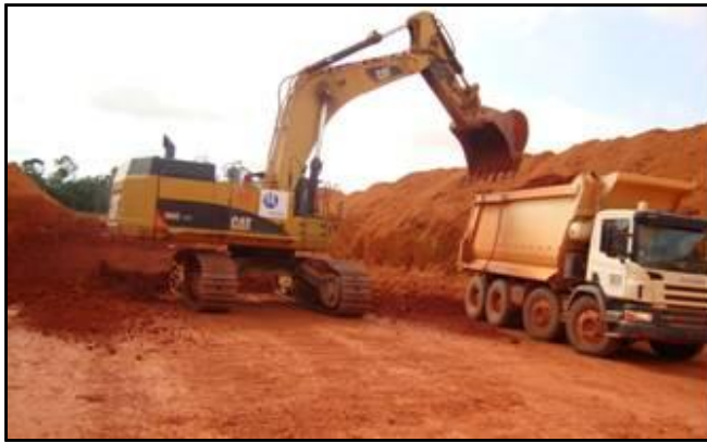
Fig 2 –Loading of ore by a hydraulic excavator
