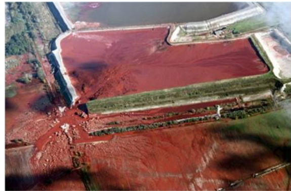
Fig. 9 Aerial photo of the Reservoir No. 10 after the dam failure in October 2010 [25]
